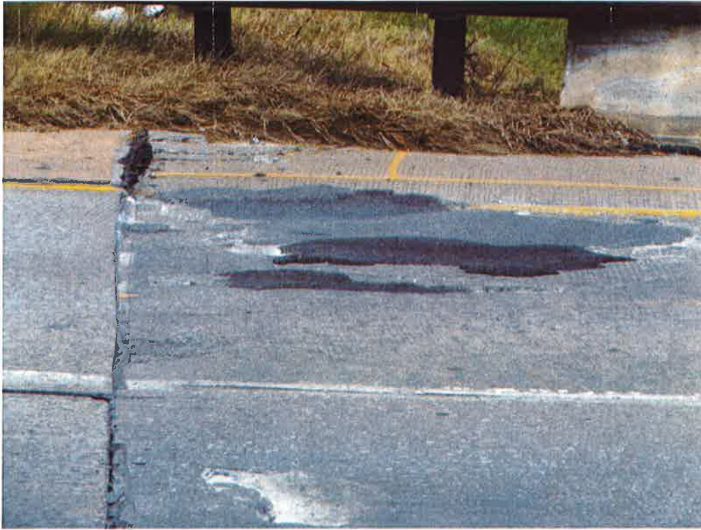
Pic # 30 Partial Depth of Approach Pavement 1
